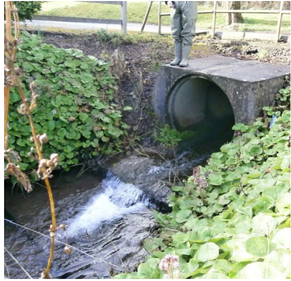
Photo 2: Existing Culvert in Woodbrook Stream (Site 1)
